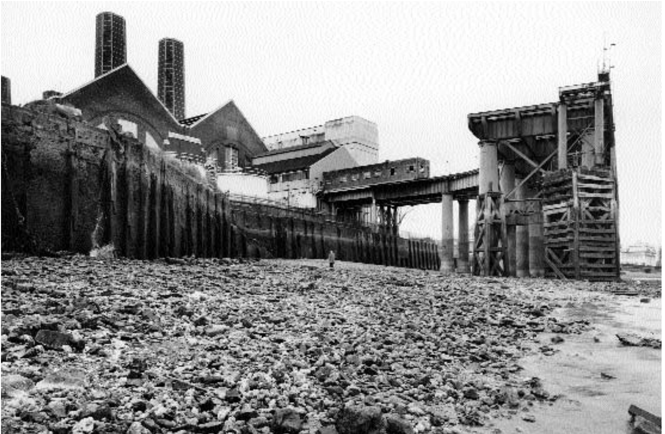
Fig. 7: Coaling jetty at Greenwich generating station
