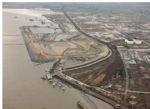
Photograph of the reclamation works (taken end January, 2011)
